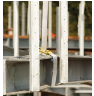
Industrial hall construction
