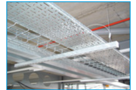
Multiple cable trays on single channel
