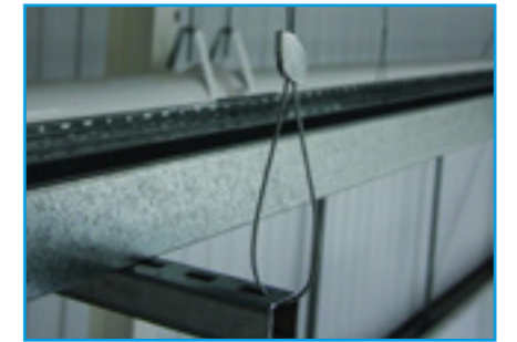
Perforated cable tray on channel
