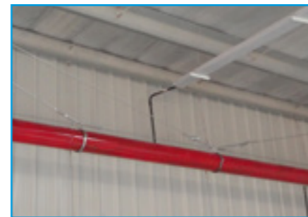
Bracing for steel pipes
