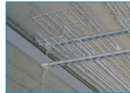
Multi-tiered cable basket on Trapeze
