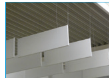
Acoustic baffles
