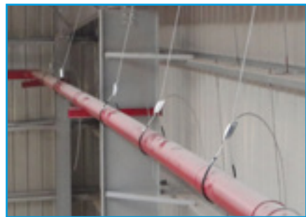
Intermediary supports for steel pipes
