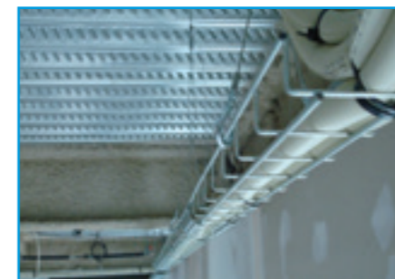
Refrigerant pipes
